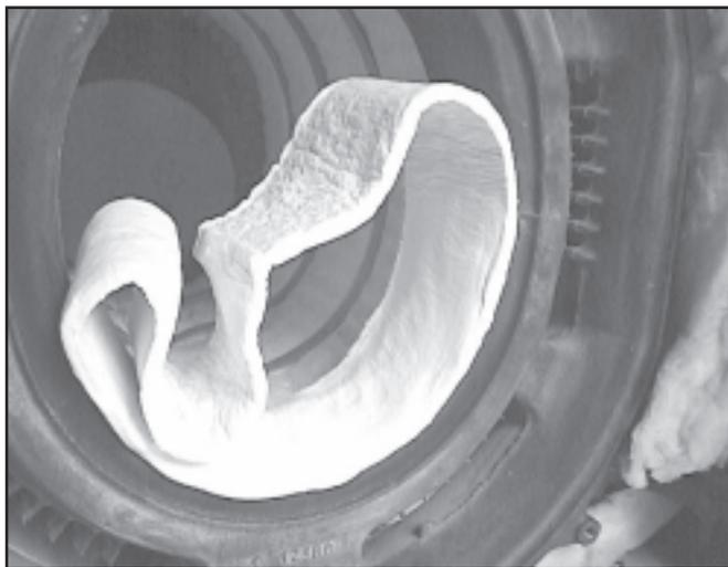
**Figure 7 - Position the "opening" liner sleeve with the outer edge even with the front opening.**
