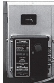
Beckett Controller with no lights and hour meter
