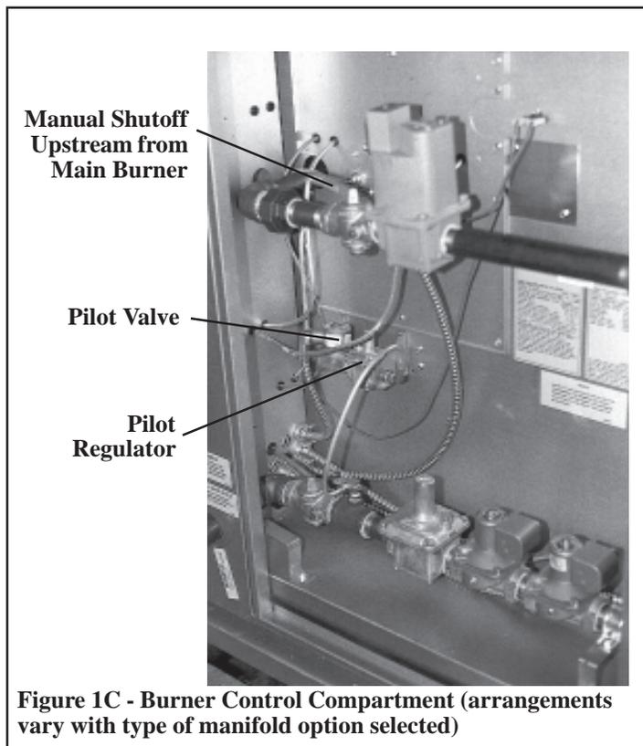
Loosen the 3/8" close nipple between the pilot regulator and the pilot valve. Remove the pilot regulator, leaving the close nipple attached to the pilot valve.
