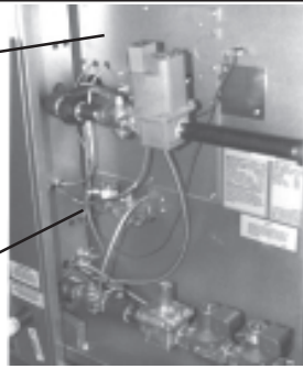
Figure 7 - Burner with the New End Plates and Hot Surface Pilot
