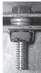
View of hanger bar hardware with heater side panel removed (for illustration only; do not remove side panel to install)
