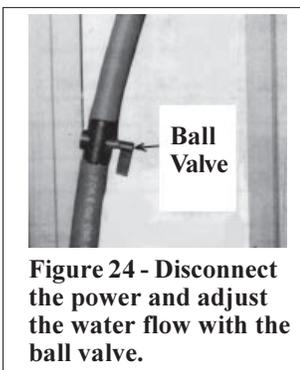
**AquaSaver® Timed Metering Control System** -- NOTE: Water flow and pad wetting time should be adjusted at maximum air flow and wet bulb depression to assure complete wetting of the media at the extreme operating conditions.
