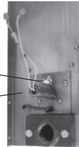
**Figure 2B - Burner End Plate of a Unit Manufactured before 3/96 with a Spark Ignition System**
