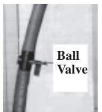
utes with the blower in operation, the water should have completely dampened the pads but should not be flowing off the entering side of the media. If water is flowing off the entering side of the media, turn the system off, disconnect the power, and reduce the entering water flow.
