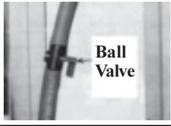
Using the ball valve, located in the middle of the length of hose running from the pump to the distribution pipe inlet, adjust the valve to allow the flow to completely dampen the media pads from top to bottom. Operate the unit watching the water flow. After 15 minutes with the blower in operation, the water should have completely dampened the pads but should not be flowing off the entering side of the media.
